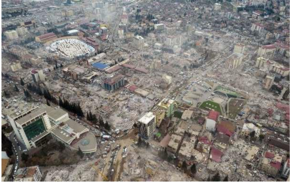
Figure 1. Devastation caused by the 7.7 and 7.6 magnitude twin earthquakes centered in Kahramanmaraş, Türkiye, on February 6, 2023 ( Kahramanmaraş Depreminin Kendine Has Özellikleri | EkoAvrasya Vakfı , 2026).
